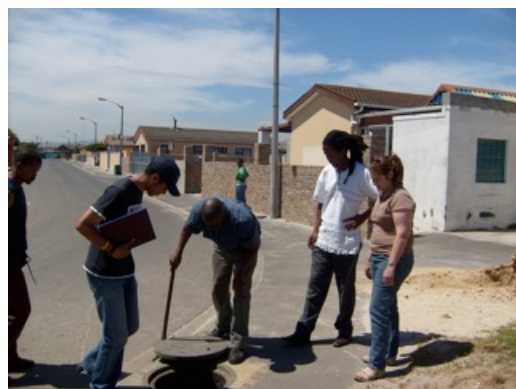
Opening of sewer
