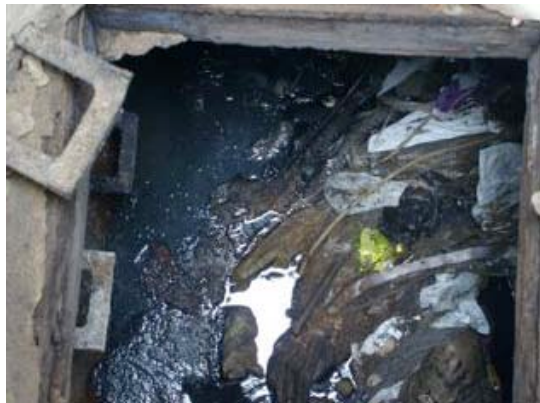
Inside the man-hole
