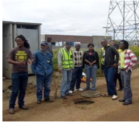
Opening the manhole
