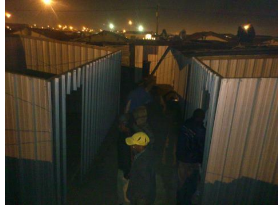
Picture 2: New shacks being constructed
